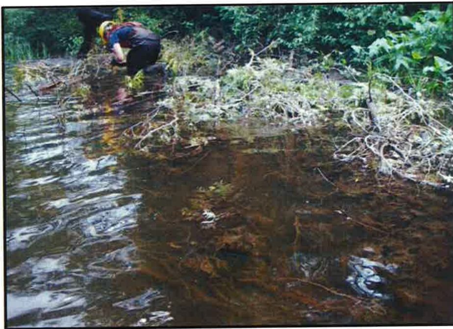
Photo 26 cedar bundles added to existing deflector at Capital Paving property
