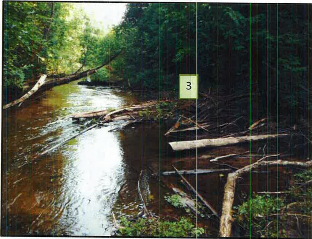
Photo 24 structure 3 deflecting thalweg
