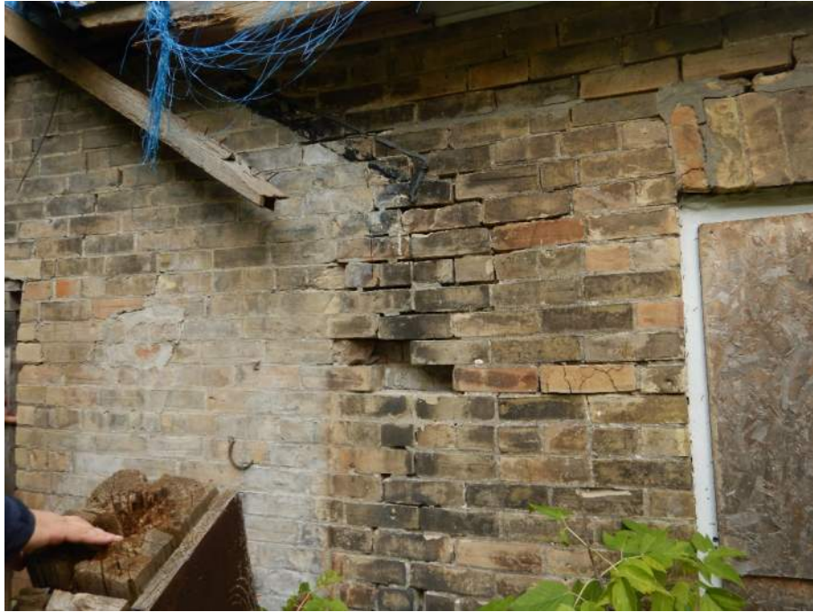
Figure 12 – Deteriorated Bricks and Mortar
