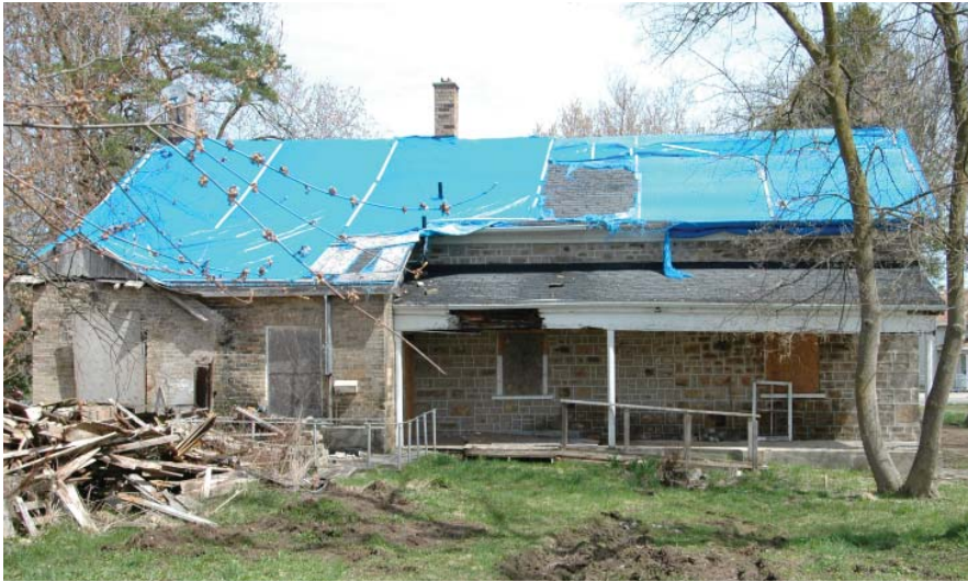
Figure 21 - Rear View of brick addition and deteriorating porch and roof. Note partial removal of yellow brick addition. Photos from site visit, January 2017.
