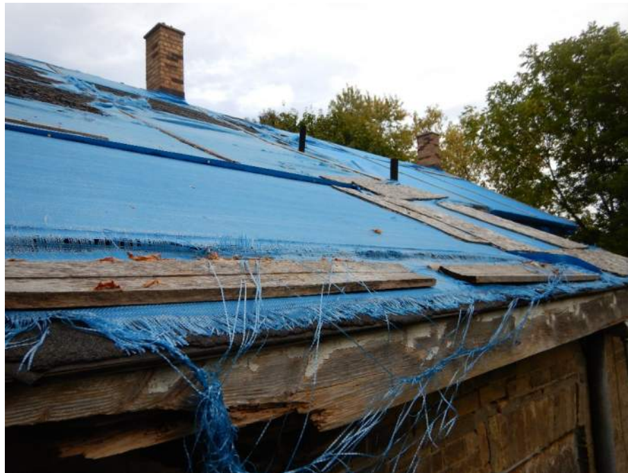
Figure 14 – Ripped Tarp on the Roof
