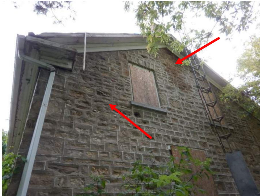
Figure 10 – Moisture on Stone Wall near Chimney
