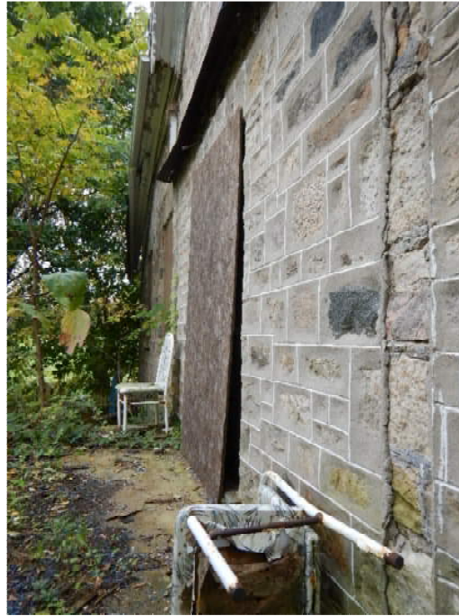
Figure 9 – Front Door Boarding Loose
