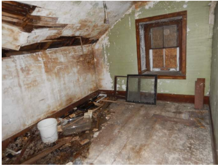
Figure 15 – Deteriorated Rafters
