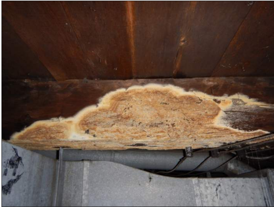
Figure 3 – Mold on Floor Beam
