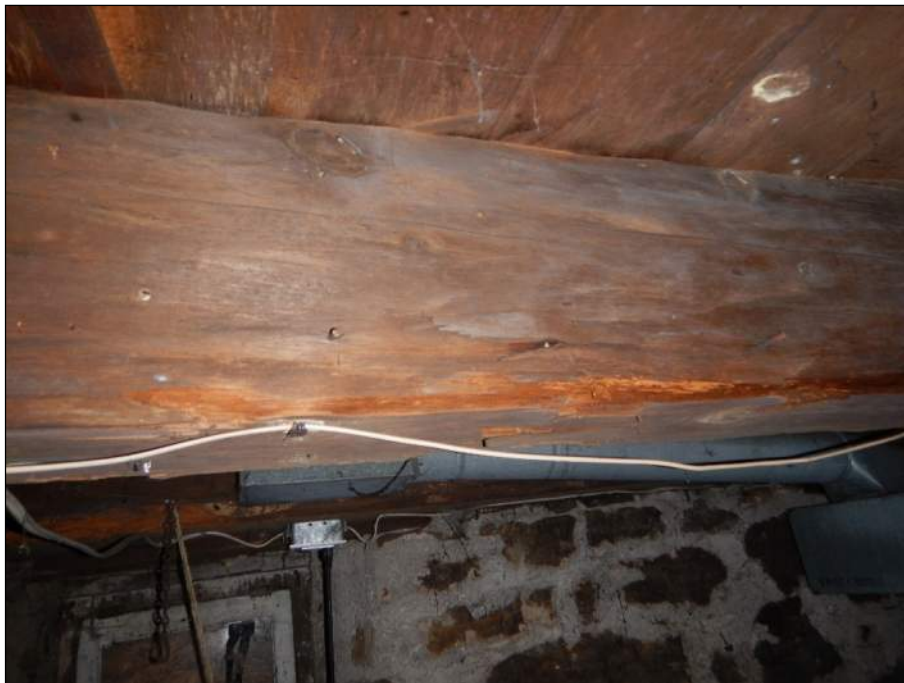
Figure 4 – Material Loss due to Rot on Floor Beam
