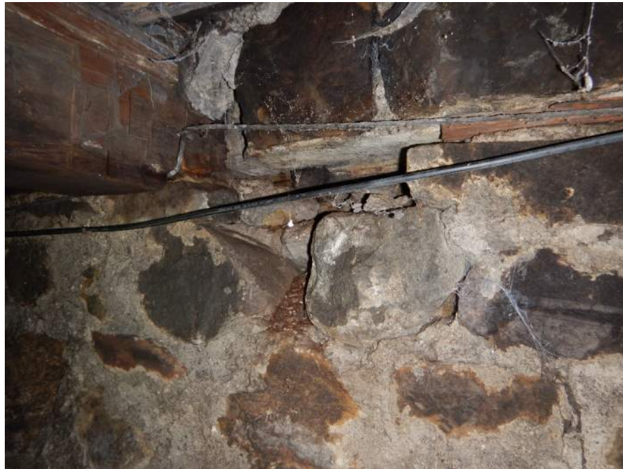
Figure 2 – Interior Mortar Deterioration
