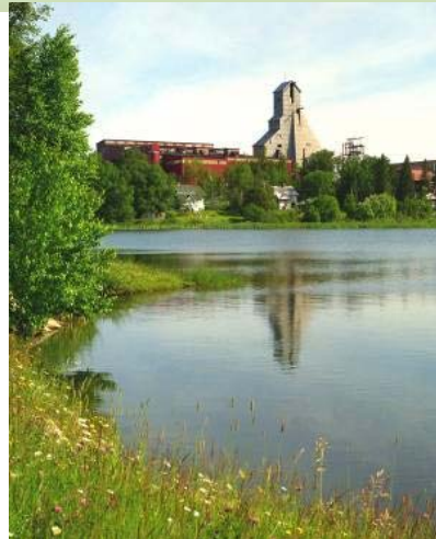
McIntyre Headframe, Timmins
