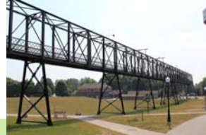
Palmerston Pedestrian Bridge Town of Minto
