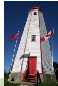
Port Burwell Lighthouse Bayham
