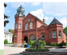
Clinton Carnegie Library
