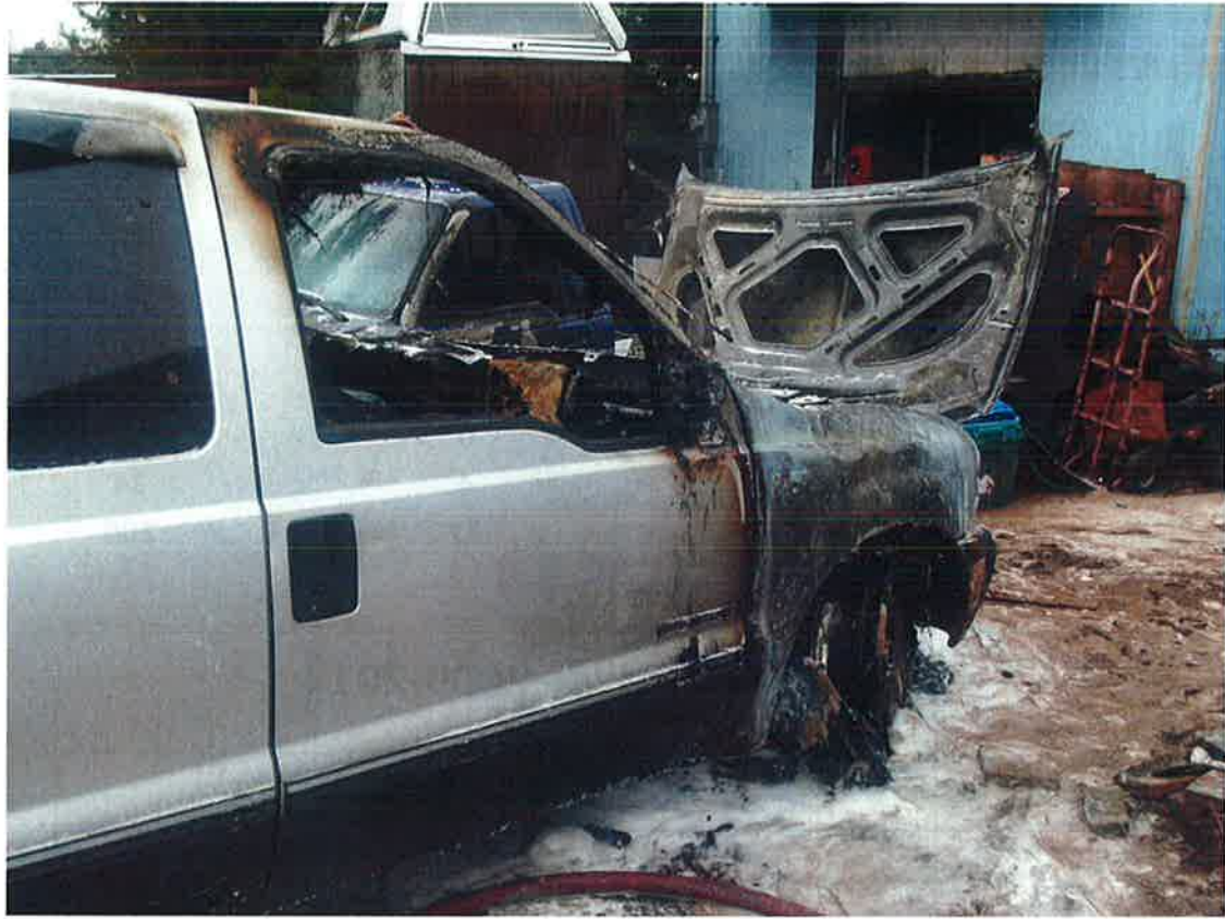
Two Vehicles and House Damaged by Fire December 27, 2014
