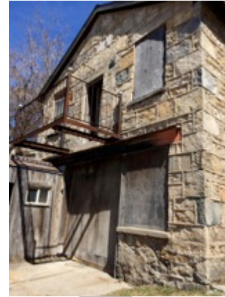
Figure 16: There are some vacant buildings in need of maintenance and repair.
