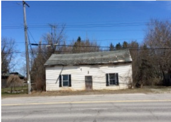
Figure 8: Some properties located along Wellington Road 46 are in need of maintenance and improvement and exhibit poor visual quality.
