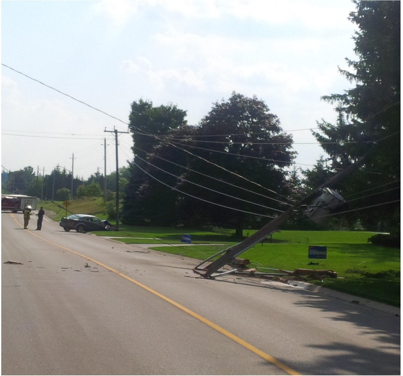
Arkell Road Motor Vehicle Collision Involving Hydro
