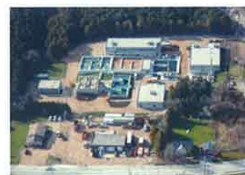
The new Elora wastewater treatment plant will improve river water quality for the world-class brown trout tailwater fishery
