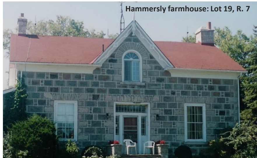
Edinburgh-coursing of fieldstones with H-PATTERN CONNECTORS made of limestone (below) and granite (right)
