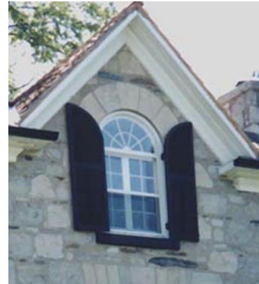
1860 former Becker store, Crieff arched gable window
