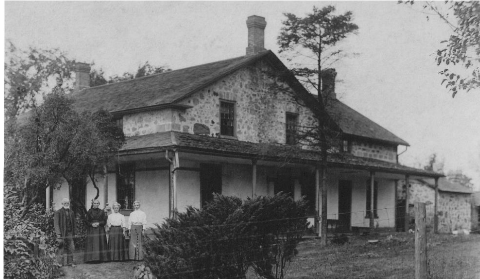
Rubblestone masonry, whitewashed under the porch where the farm workers washed up before entering the kitchen, reflects Waterloo County architectural style.
