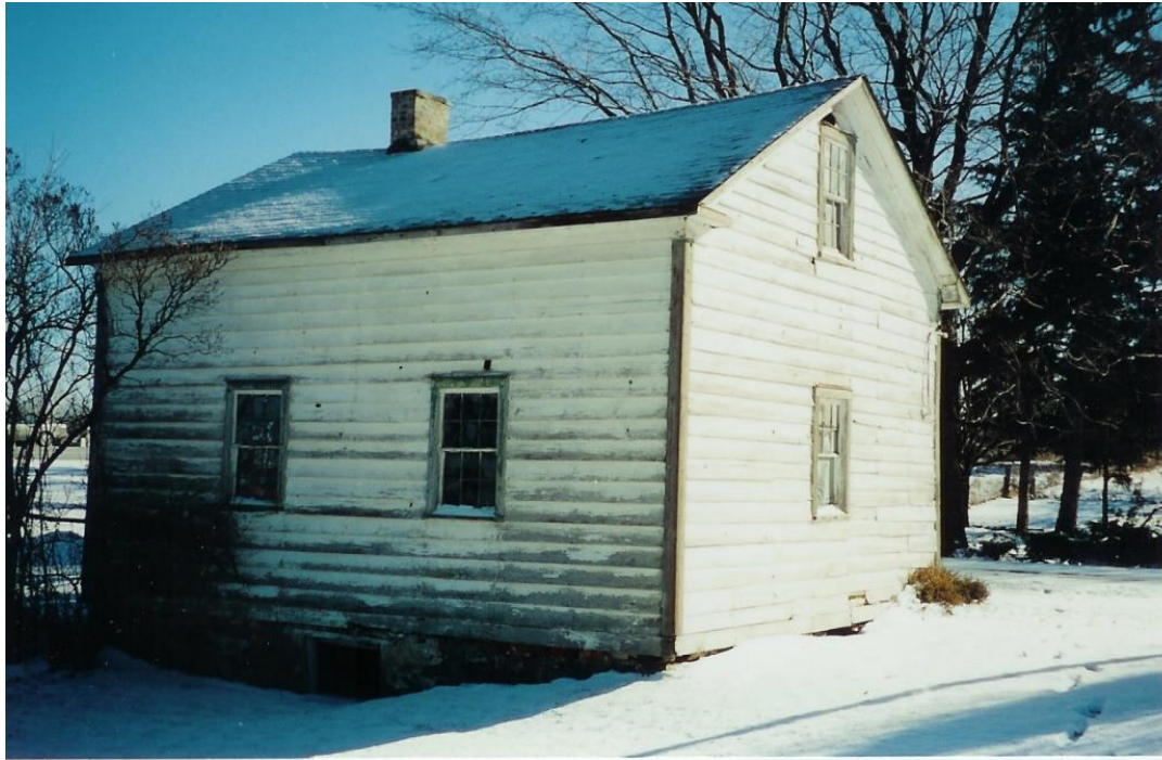
1829 Winer Family's Cedar Log Dwelling Ship's-lap siding was added over a century ago to protect the logs and cut down drafts.
