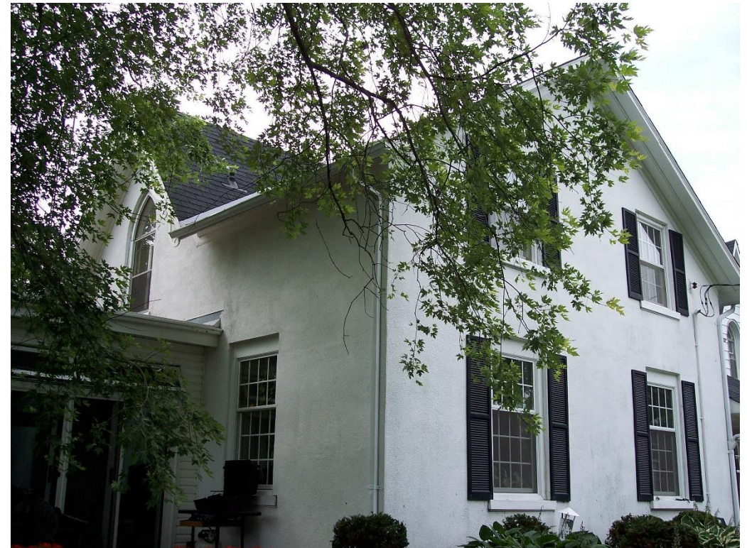
Barrett farmhouse, lot 5 R. Conc. 2, has stucco facing .
