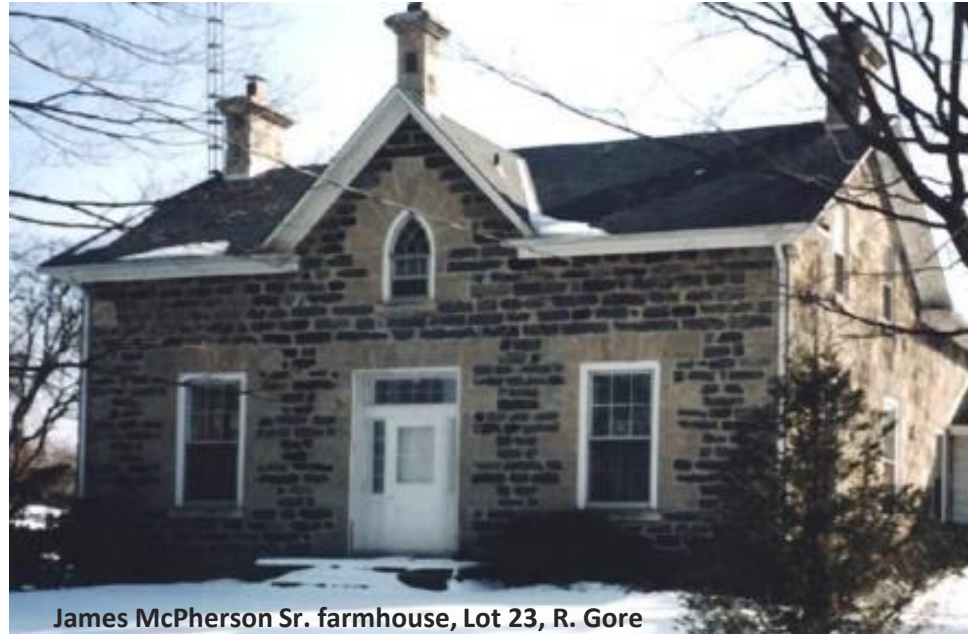
Straight-coursed granite, with limestone quoins, and voussoirs over gable window (below).
