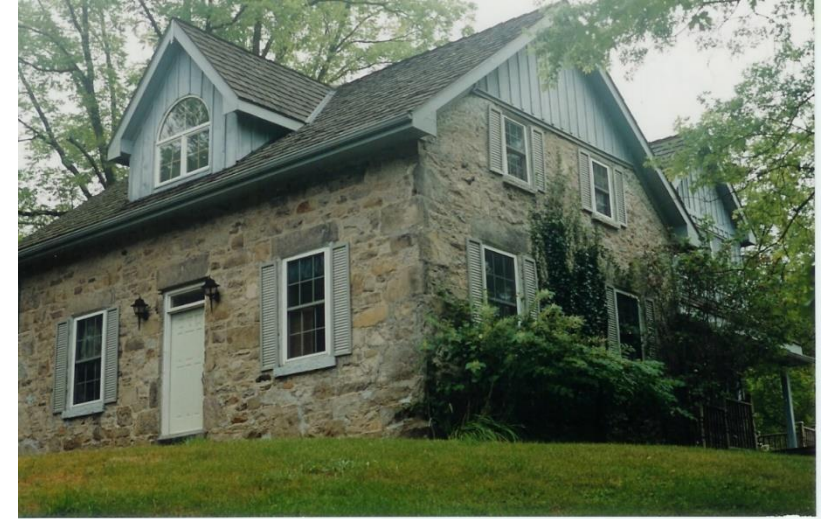
Johnston house, E. side Brock Rd., Lot 18 F. 8
