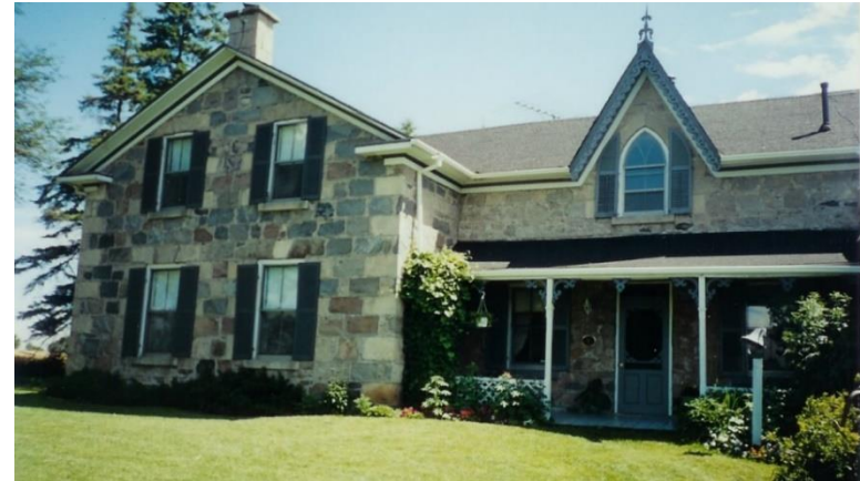
Side view of Hector McCaig farmhouse showing kitchen wing.
