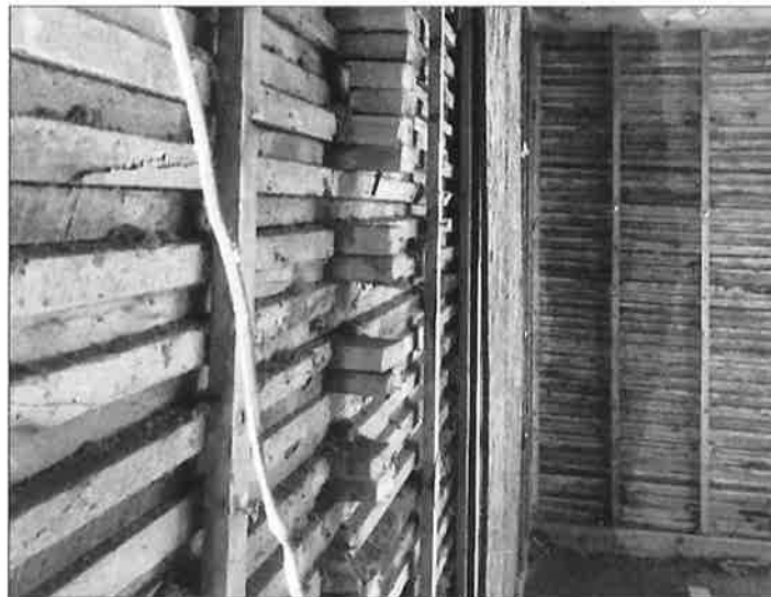
Interior view showing the offsetting of the planks to receive plaster, and remnants of former plank-on-plank partitions. (City of Markham, 2018)
