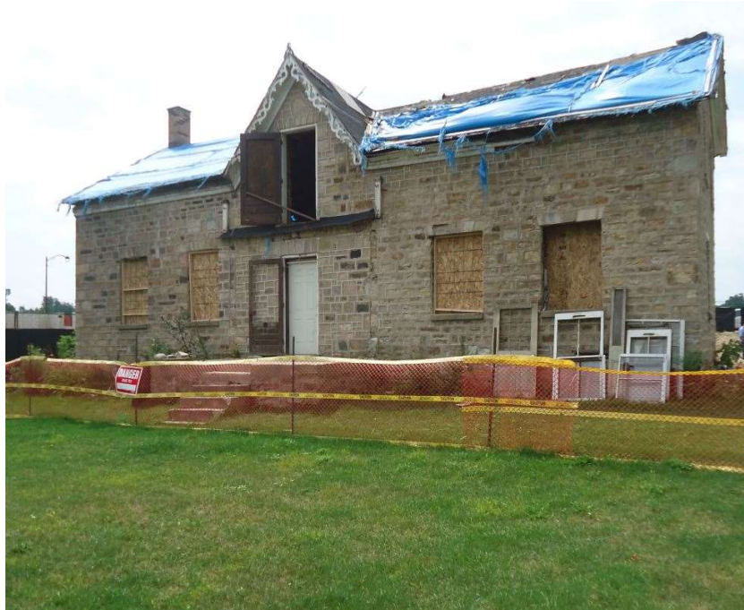
Photo 1: Front elevation, viewed from Brock Road S.
