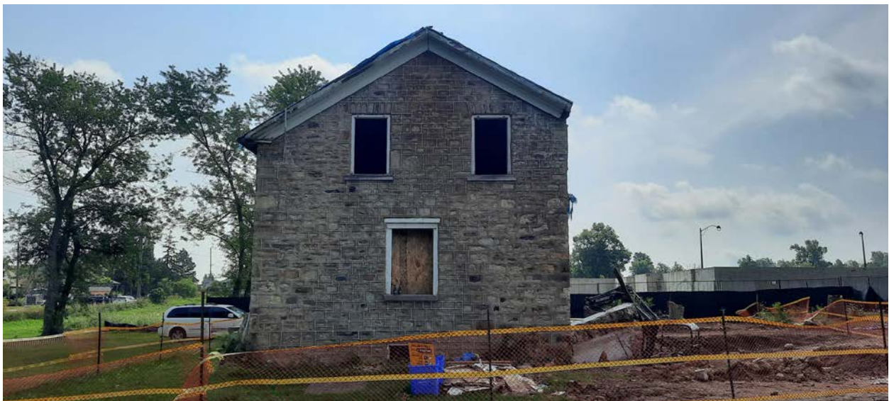
Figure 4 CBO photo of exterior taken August 11, 2021
