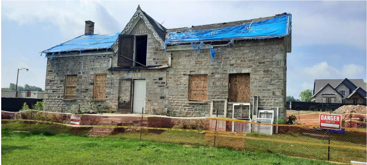
Figure 3 CBO photo of exterior taken August 11, 2021
