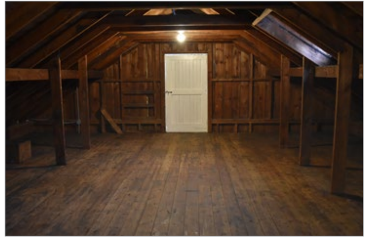
Interior attic space.
