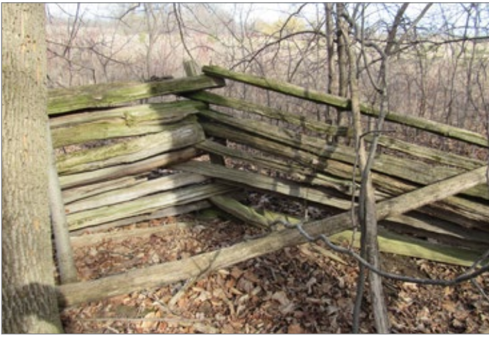
An intact section of the same snake rail fence, eight rails high. (G. Duncan, 2021)
