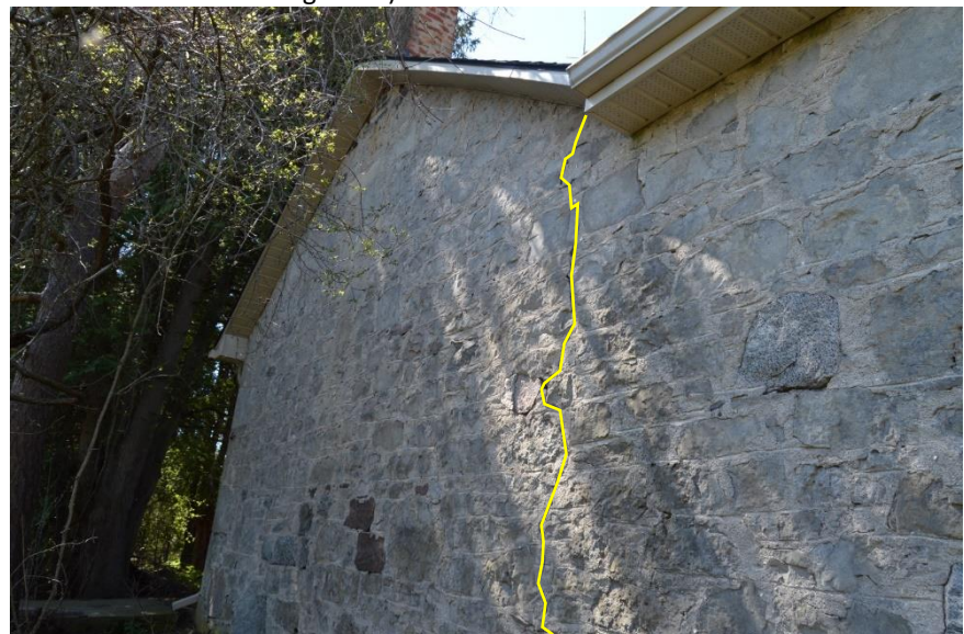
Back Wing's East Elevation – at south end showing an old vertical crack
