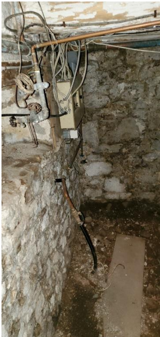
Missing Water Meter, open end pipe
