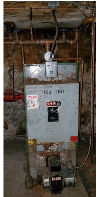
Oil-Fired Boiler
