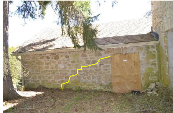
Back Wing's West Elevation (the crack is filled with cement)
