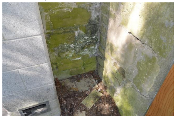
Intersection at Back wing's South Elevation and 2 Storey addition (showing the level of moss growth)
