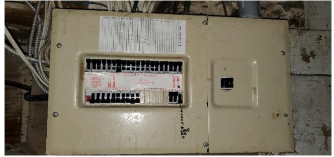
200A, 120/240V, 1-Phase Electrical Panel
