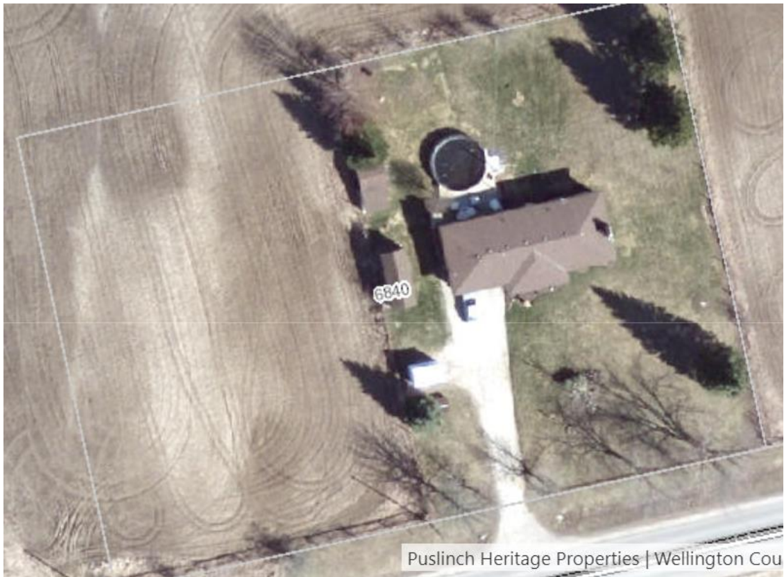
Figure 2 – Existing Conditions on Subject Property (Aerial)
