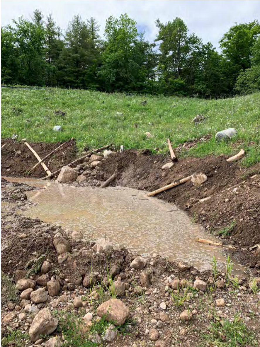
Photo 7 – View of Wetland SW1 while under construction. CRH 2022-06-09
