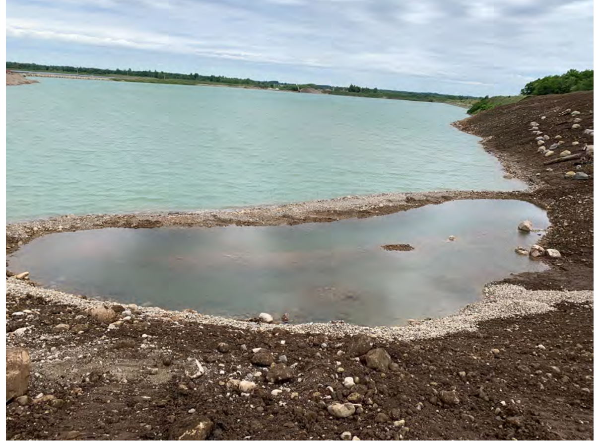
Photo 12 – View showing Wetland SW3 immediately after construction. Compare with Photos 4 and 6, showing Wetland SW3 under late season conditions in early November. SW3 has no direct surface connection with the Phase 2/6 Lake, except potentially under high water conditions. CRH 2022-06-09
