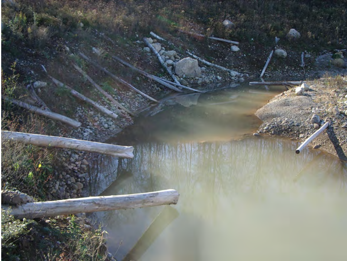
Photo 9 – View of Wetland SW1. This feature along with Wetlands SW2 and SW3 were seeded with a custom native wetland seed mix in early November 2022.
