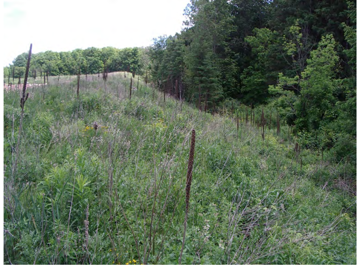
FP06a - View looking east along Unit SB1. GEC 2022-06-10
