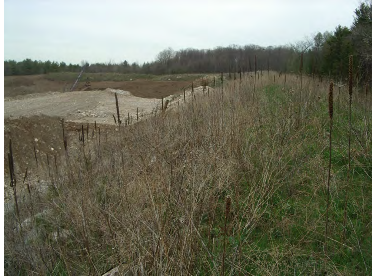
FP05a – View looking east along Unit SB1. GEC 2022-05-06
