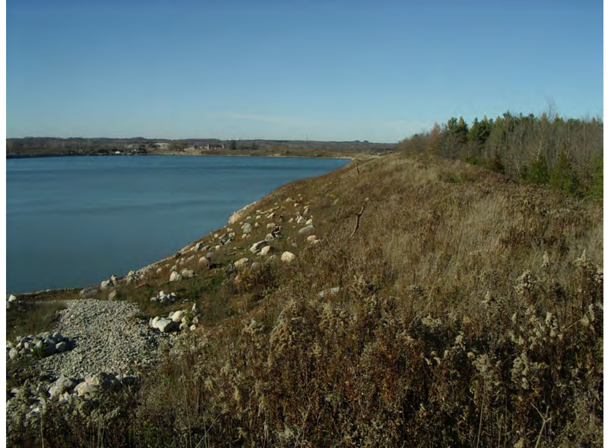
FP08a - View looking north along Unit EB1. GEC 2022-11-09
