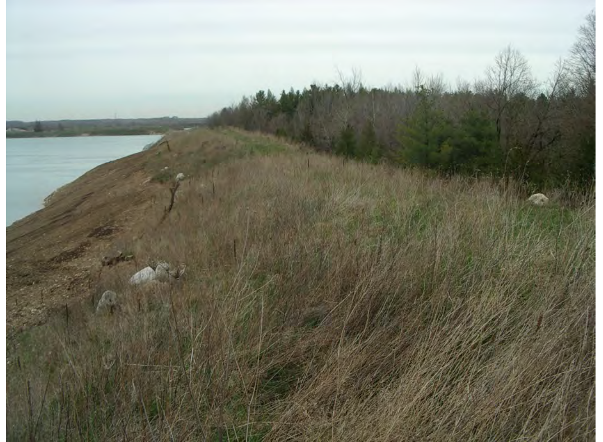
FP08a - View looking north along Unit EB1. GEC 2022-05-06
