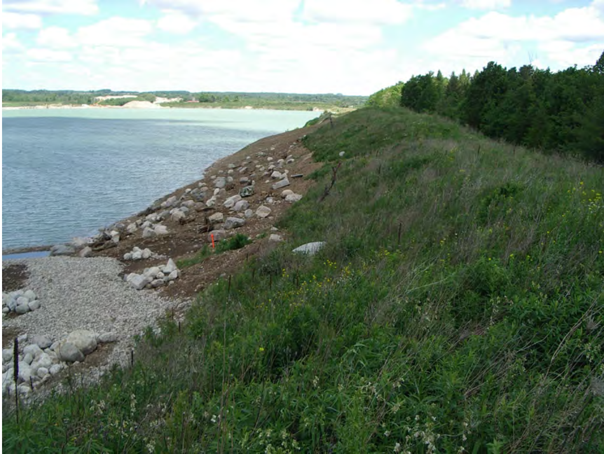
FP08a - View looking north along Unit EB1. GEC 2022-06-10
