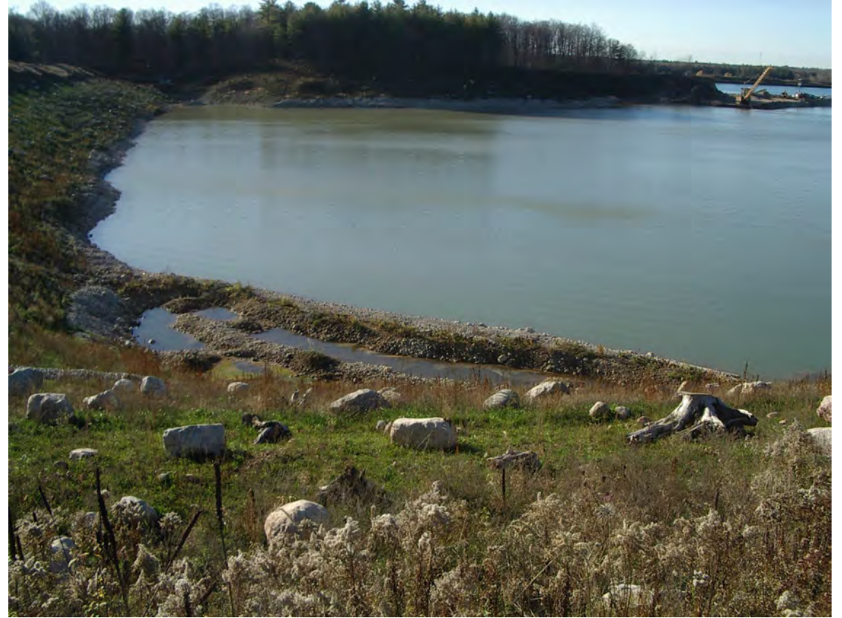
Photo 4 - View looking west northwest towards Rehab Slopes RSW1 and RSW2. Below water table extraction continues, as the Phase 2/6 Lake expands in size. GEC 2022-11-09
