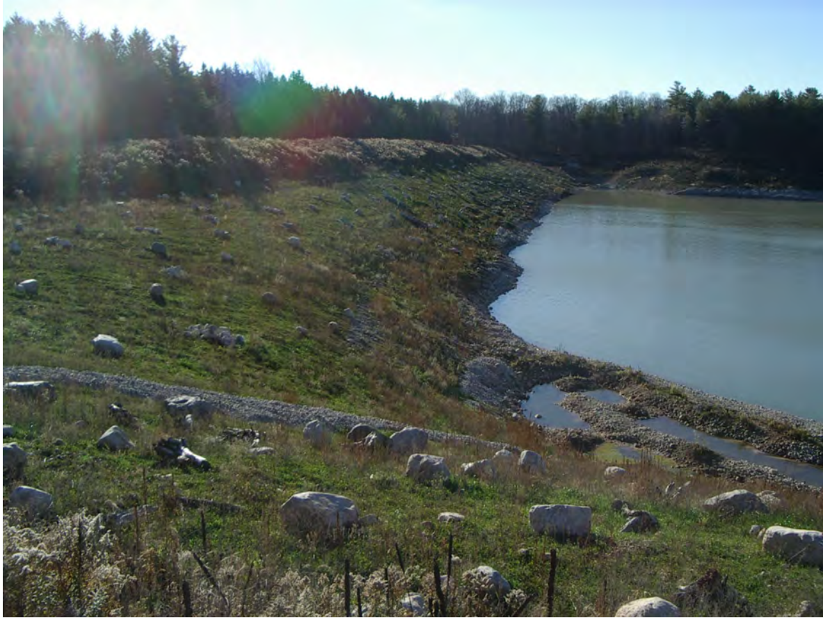
Photo 3 - View looking west along Rehab Slope RSW3. Newly-created Wetland SW3 is in the lower right. GEC 2022-11-09
