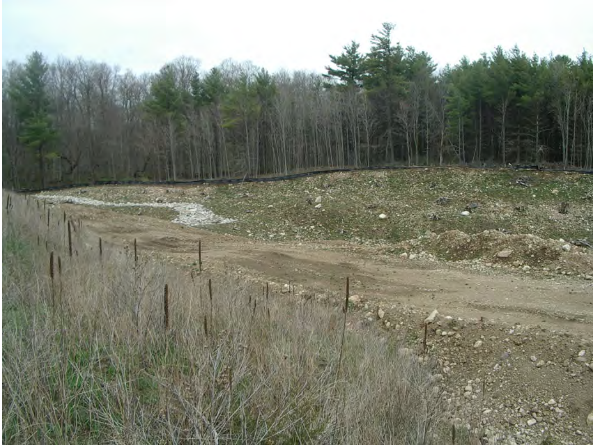
FP05c - View looking west northwest towards Woodland Protection Zone 'B' and Unit RSW2. Panorama - Left - GEC 2022-05-06
