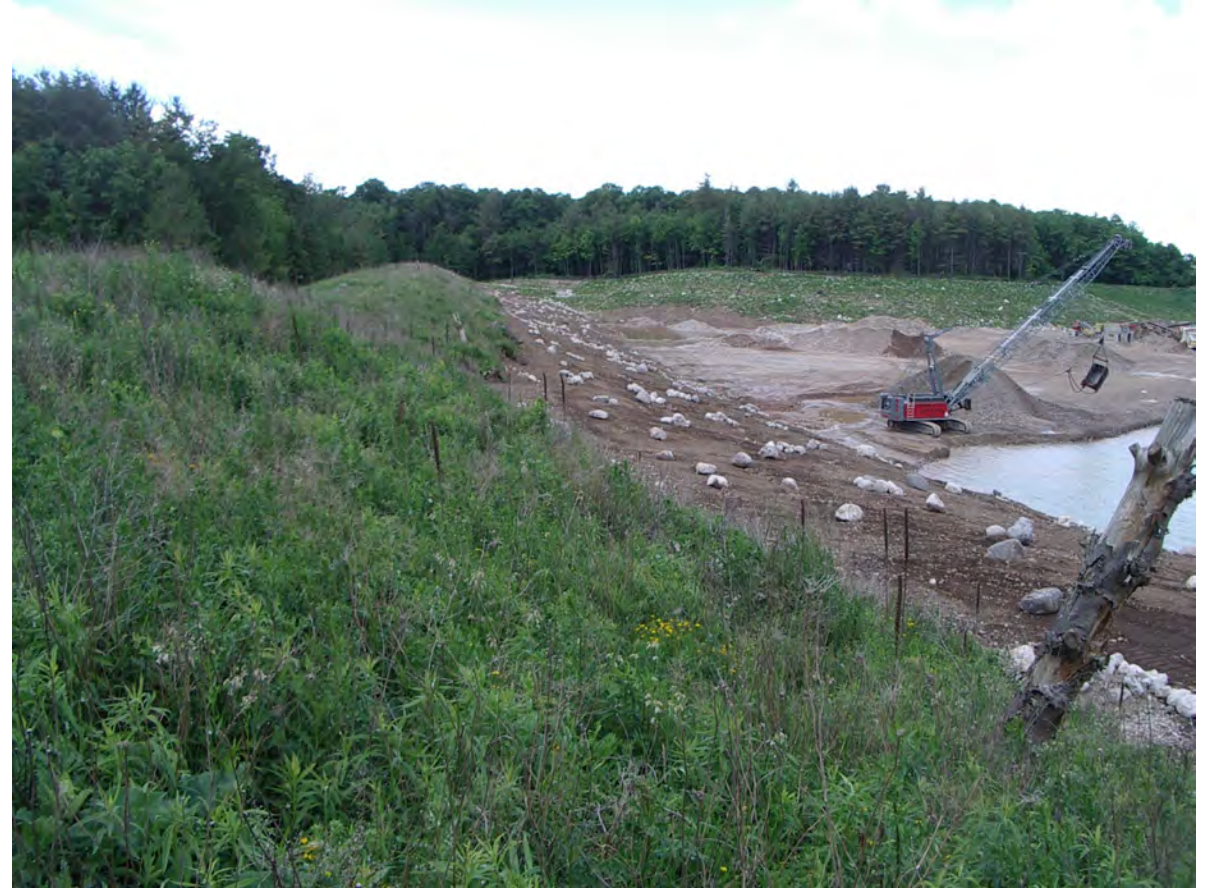
FP08b - View looking west along Unit SB1. GEC 2022-06-10
