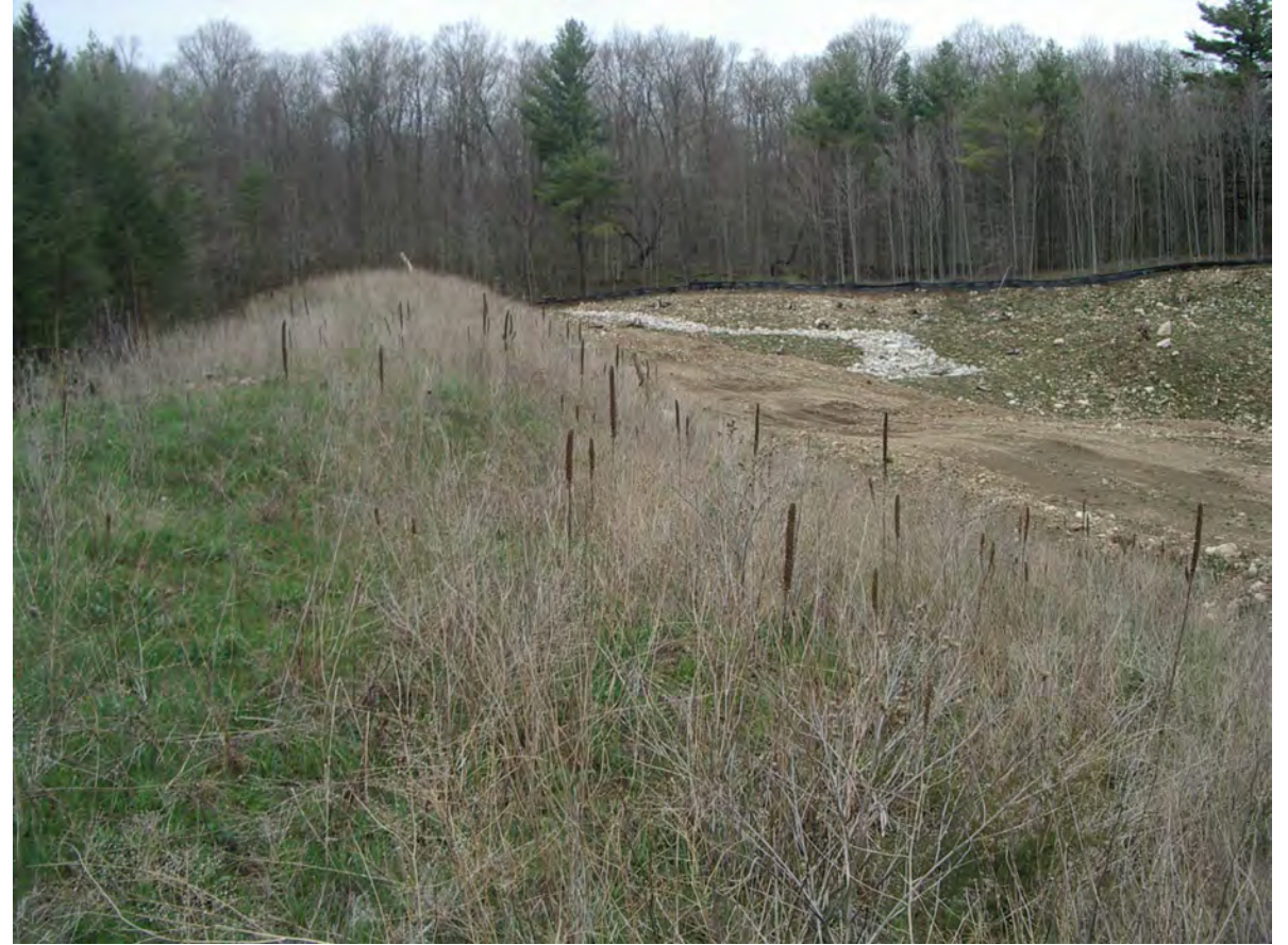
FP05b - View looking west along Unit SB1. GEC 2022-05-06
