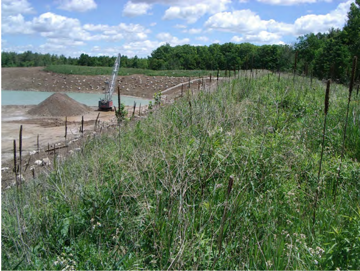
FP05a – View looking east along Unit SB1. GEC 2022-06-10
