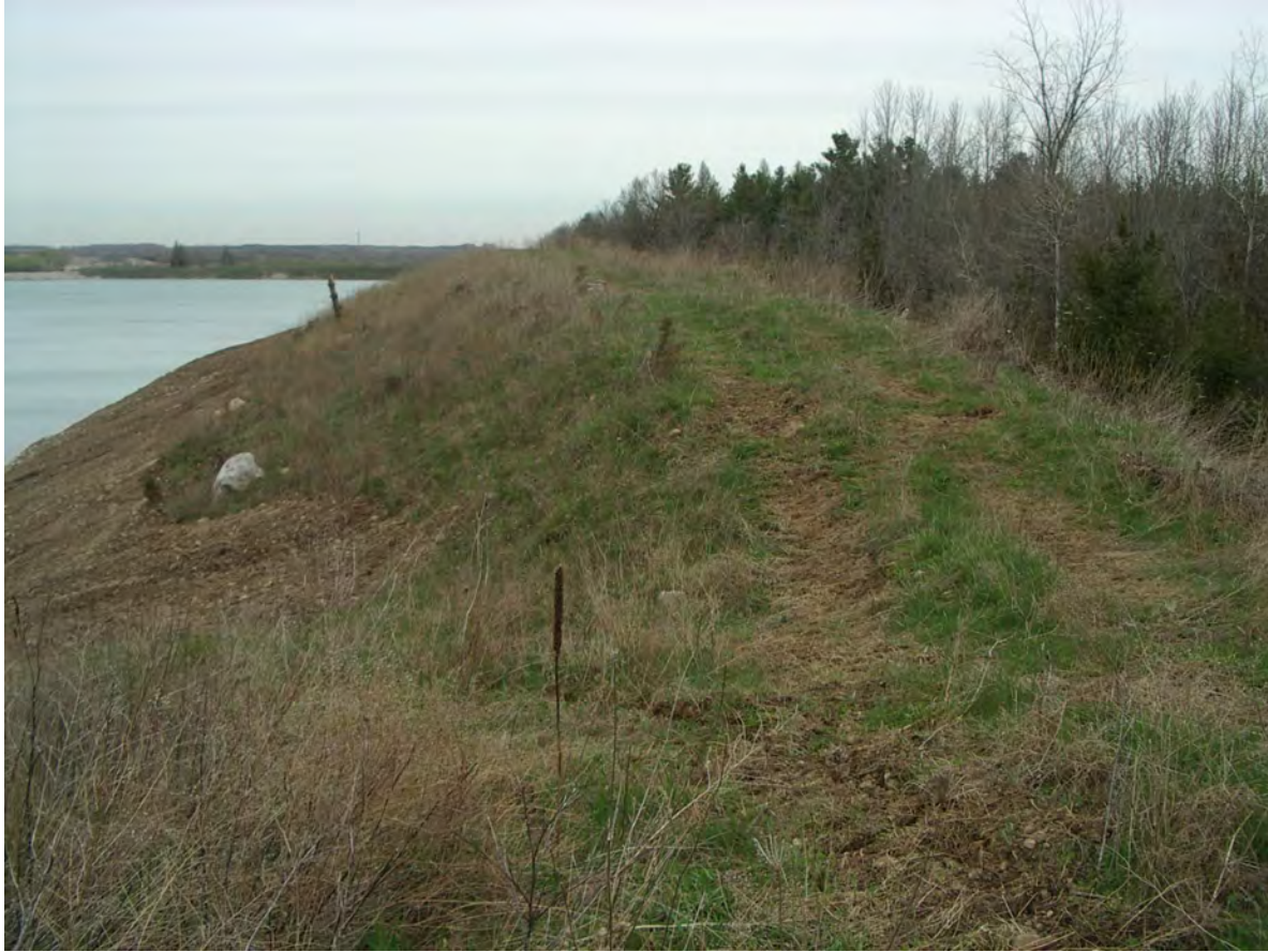
FP10a - View looking north along Unit EB1 and towards Unit EB2. GEC 2022-05-06
