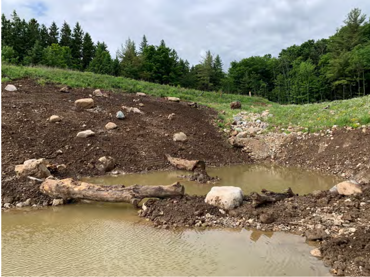
Photo 11 – View showing Wetland SW2 immediately after construction. Rocks and logs were used to create habitat features. Note the open connection with the Phase 2/6 Lake. CRH 2022-06-09
