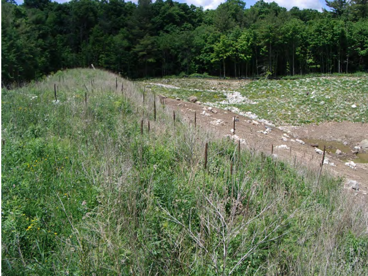
FP05b – View looking west along Unit SB1. GEC 2022-06-10
