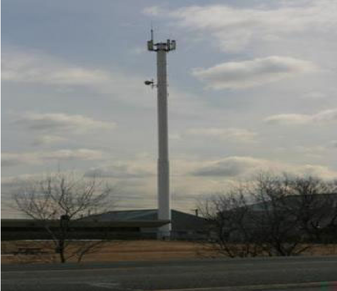
Figure 2- Example of Flush Mount Monopole (Type FM)
