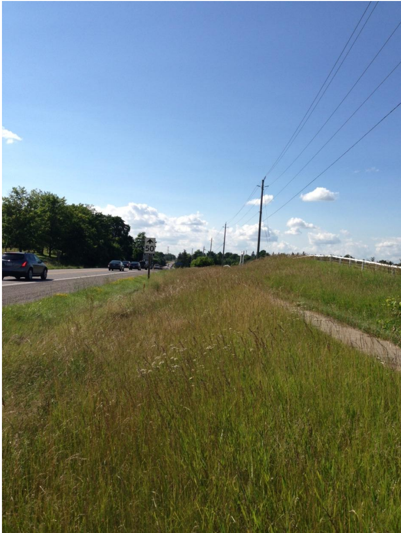
View to north along the east side of Highway 6 from the residence at 107 Queen Street.
