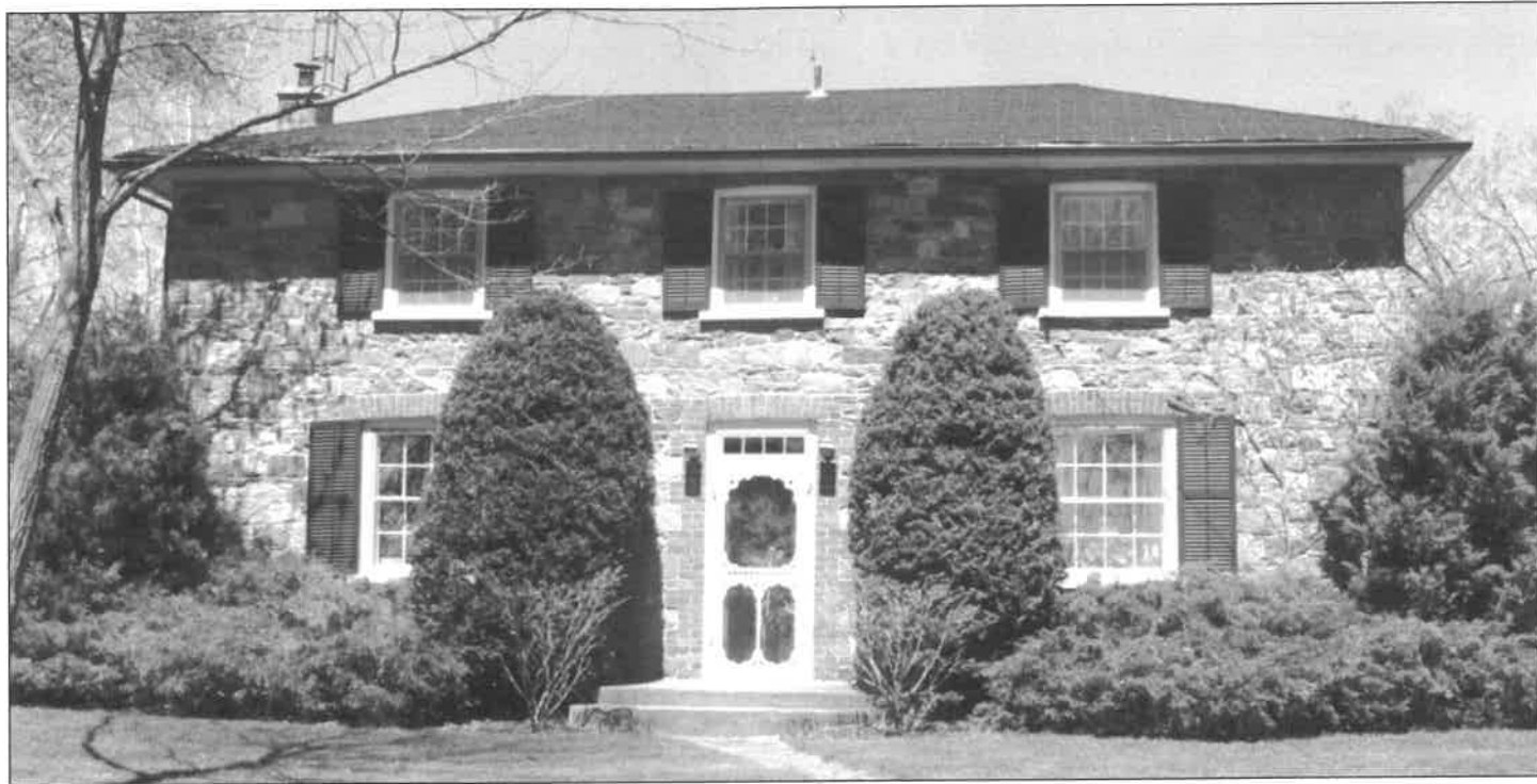
The English origin of Joseph Graham, the original owner of the Graham-Hallman House in north-east Markham, is evident in its design. The house was constructed c.1850 of local field stone trimmed with red brick and is in an excellent state of preservation. Designation under Part IV of the Ontario Heritage Act is in progress. (Photo courtesy of the City of Markham)
