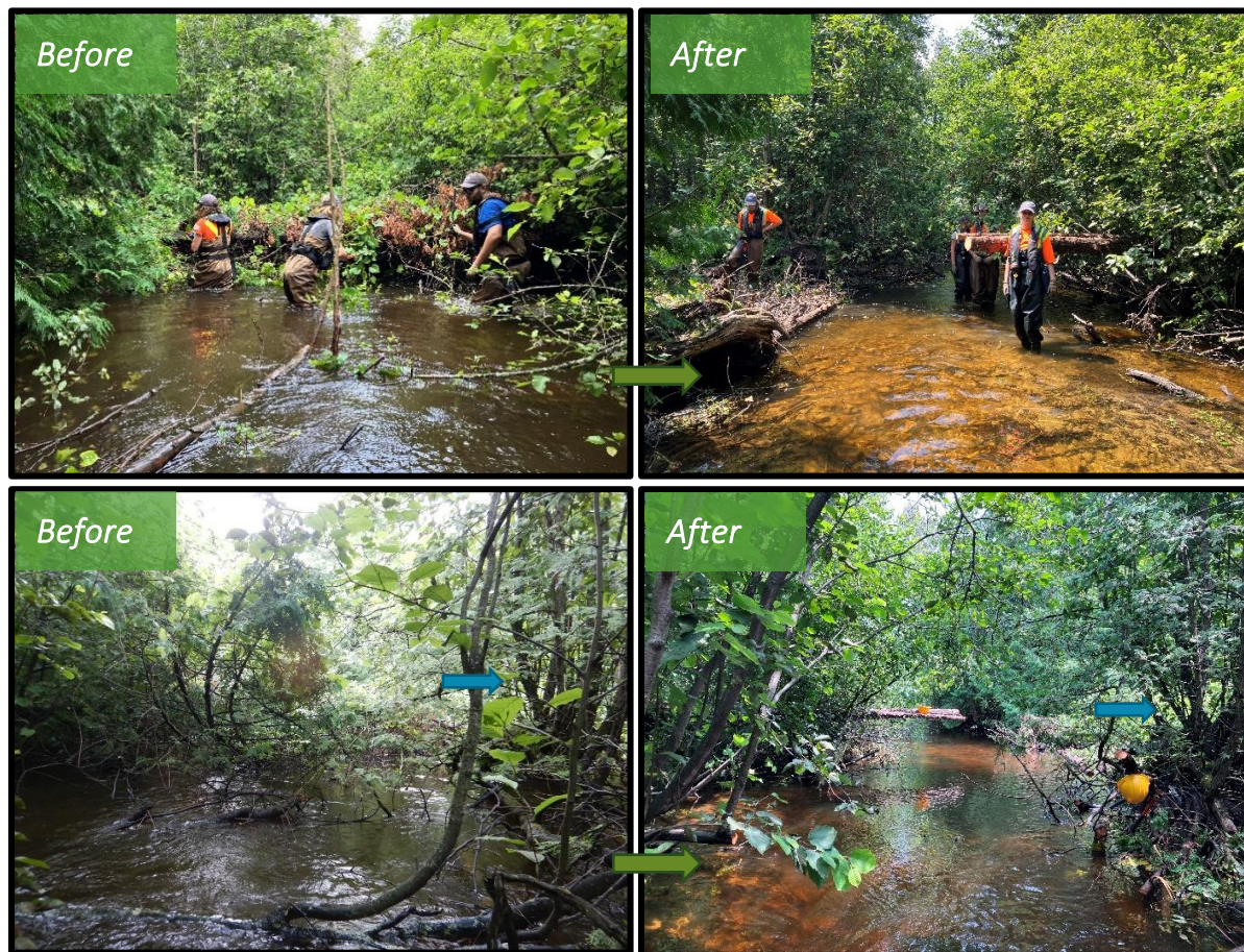
Figure 11: Before and after photos of major log jams in a series extending over 17.9m of stream
