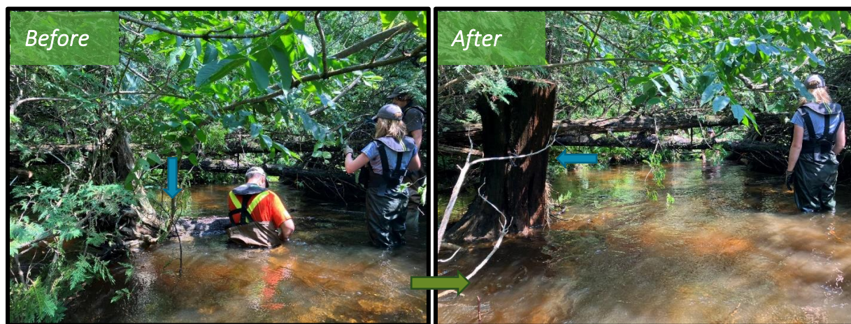
Figure 12: Shahdad sawing a large stump with root ball still attached (left). Stump upturned and stabilized to create fish habitat in the underwater root system and to unblock channel flow (right).
