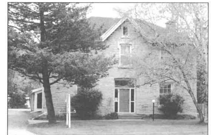
Figure 3: Peter Day House-front. (Photo by D. Taylor)
