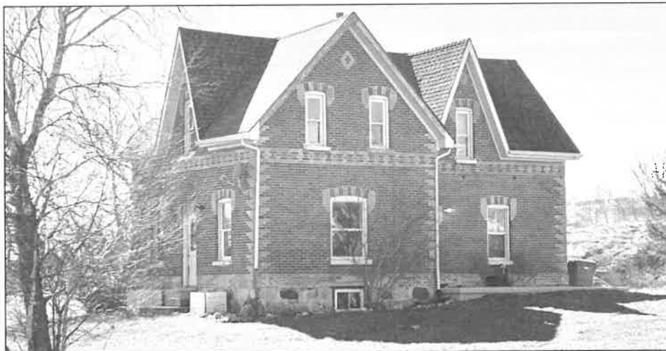
The addition is tucked behind the original house in this view of the south-east corner. (Photo by Nancy Matthews)
