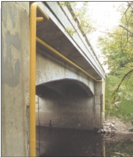
Attaching gas line on a bridge.
