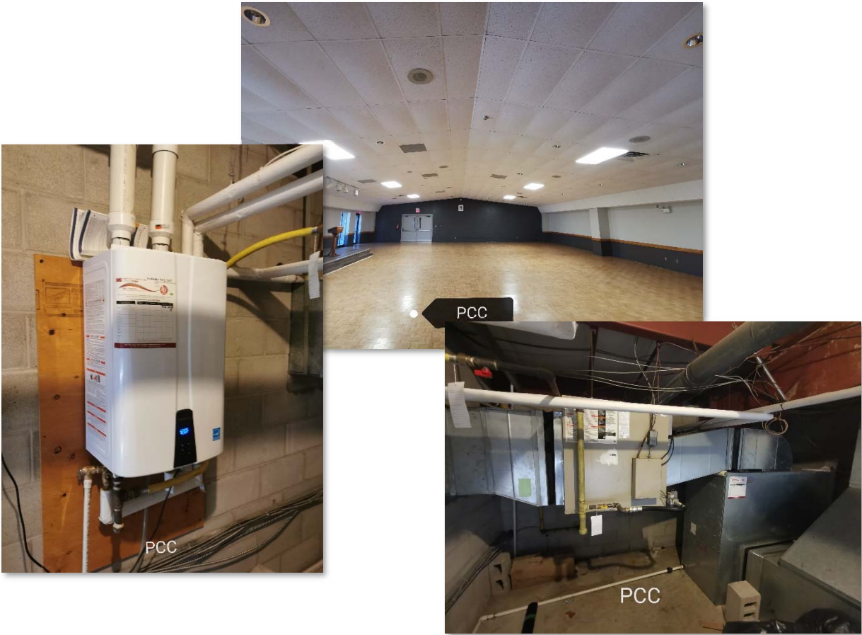
Figure 5.2 Energy Efficient Upgrades at the Puslinch Community Centre
