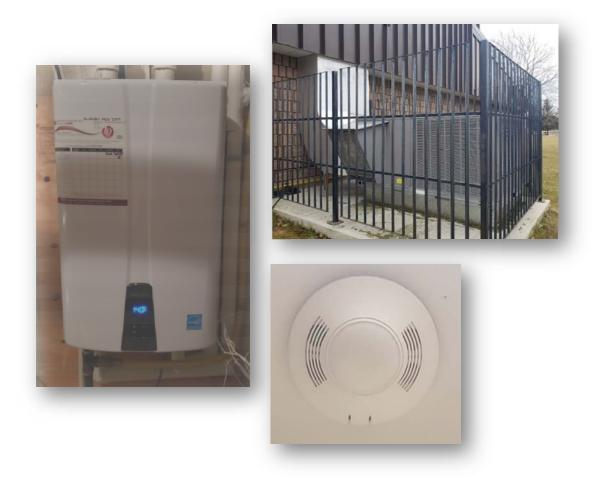
**Figure 6:** Photographs of the new high efficiency HVAC unit, instantaneous water heater and a motion sensor installed at the Community Centre.
