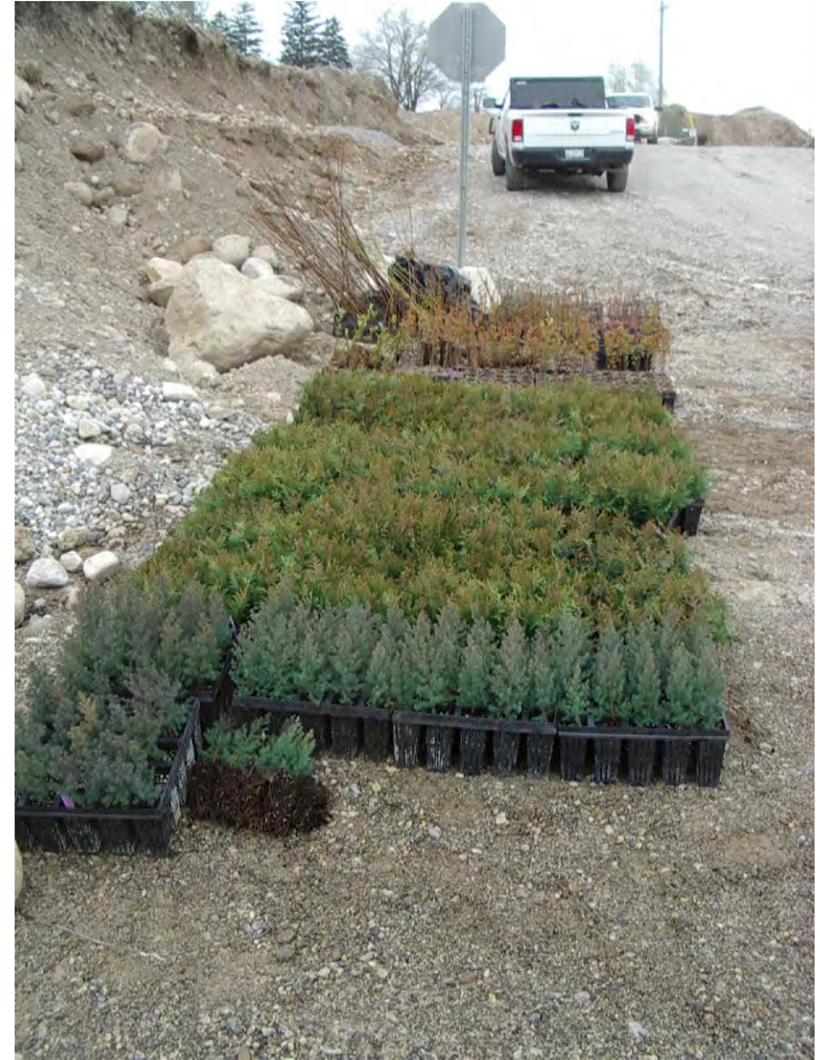
Photo 2: Plugs were selected due to the limited access and difficult terrain in Phase 6. Planting large numbers of container-grown stock was not practical. GEC 2023-04-25
