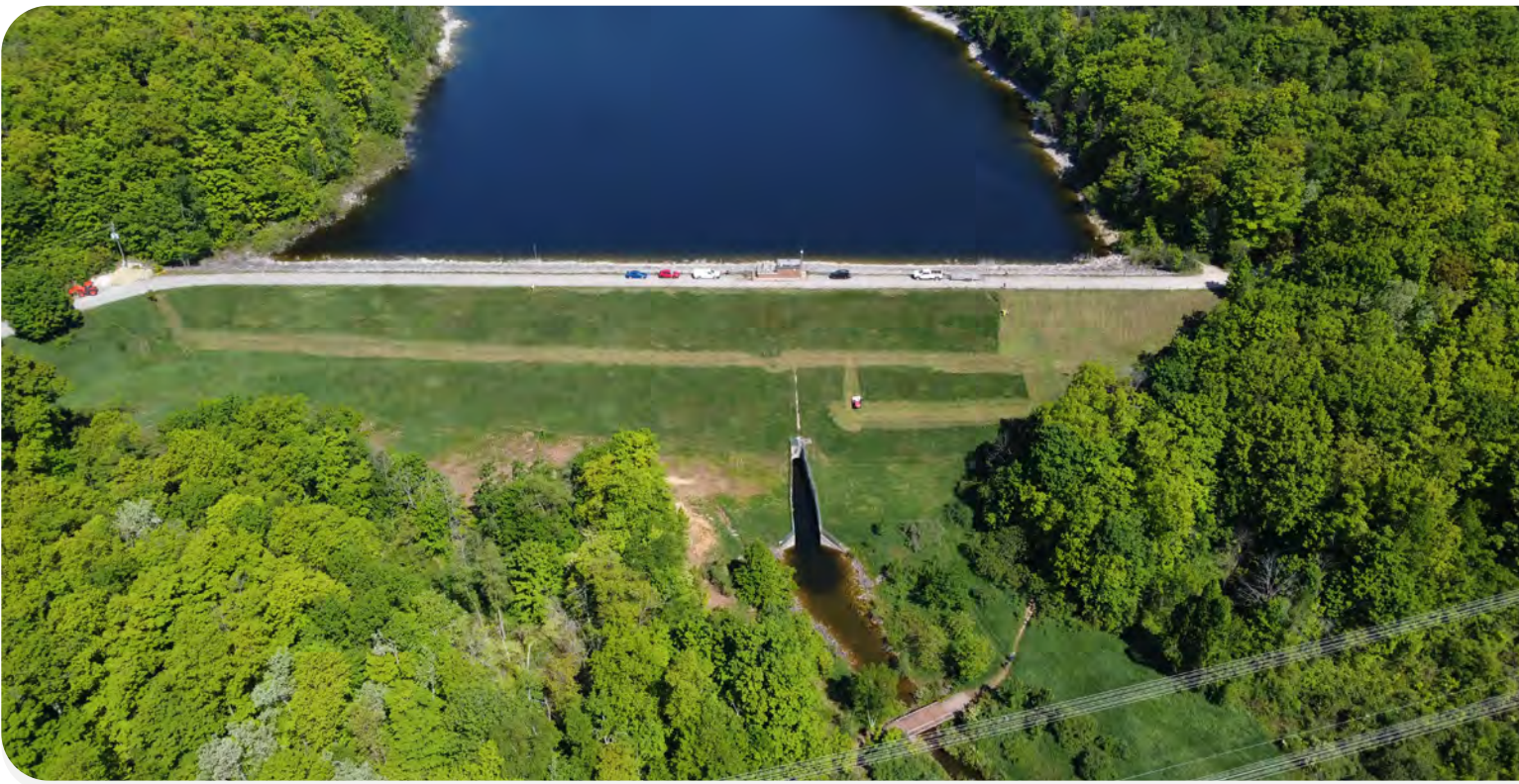
Top: Hilton Falls Dam & Reservoir
