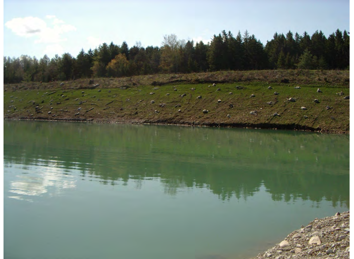
Photo 14: View looking south southeast towards rehabilitation side slope Unit RSW3. GEC 2023-04-26
