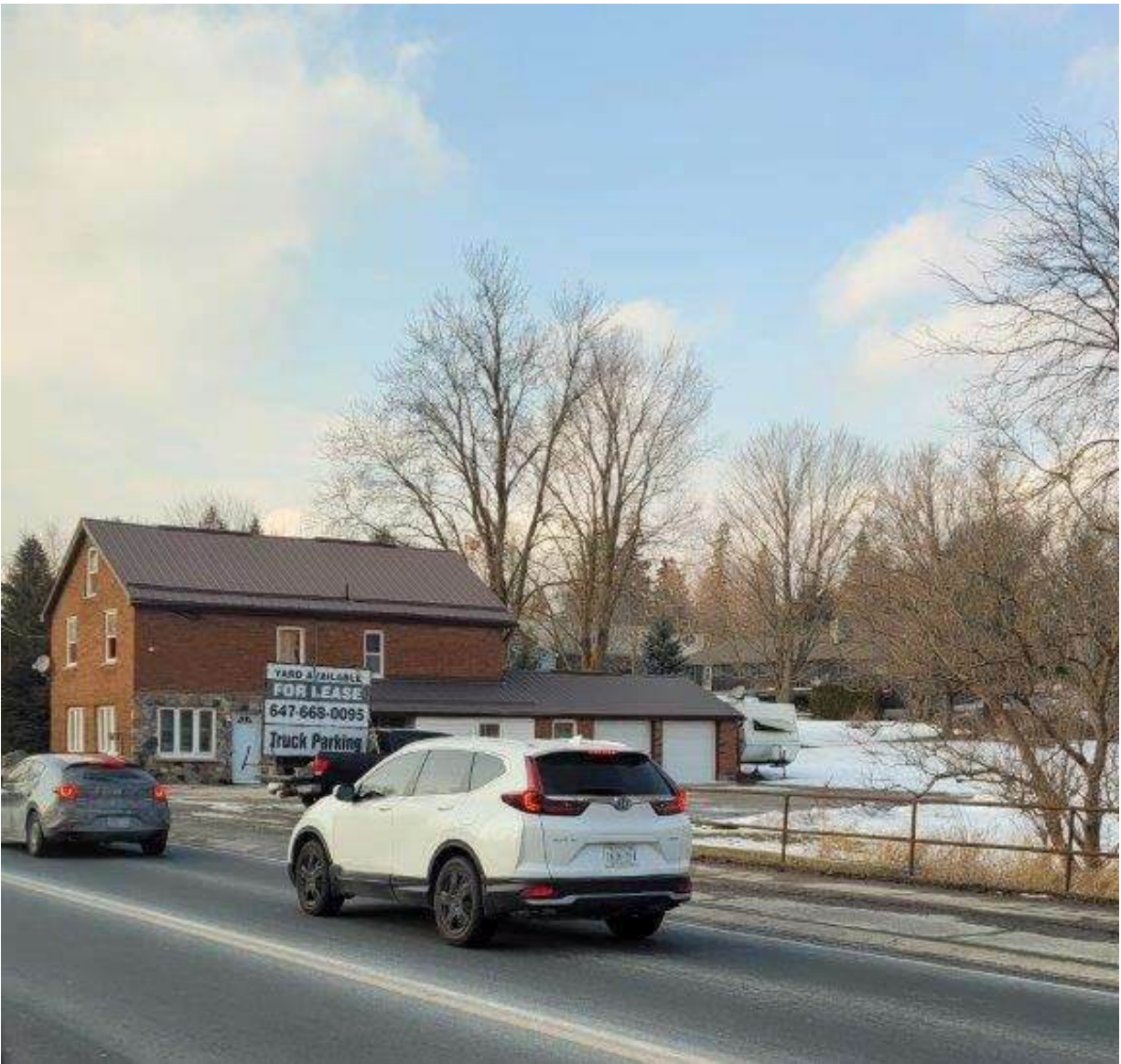
Photograph No 7. – West adjacent commercial site.
