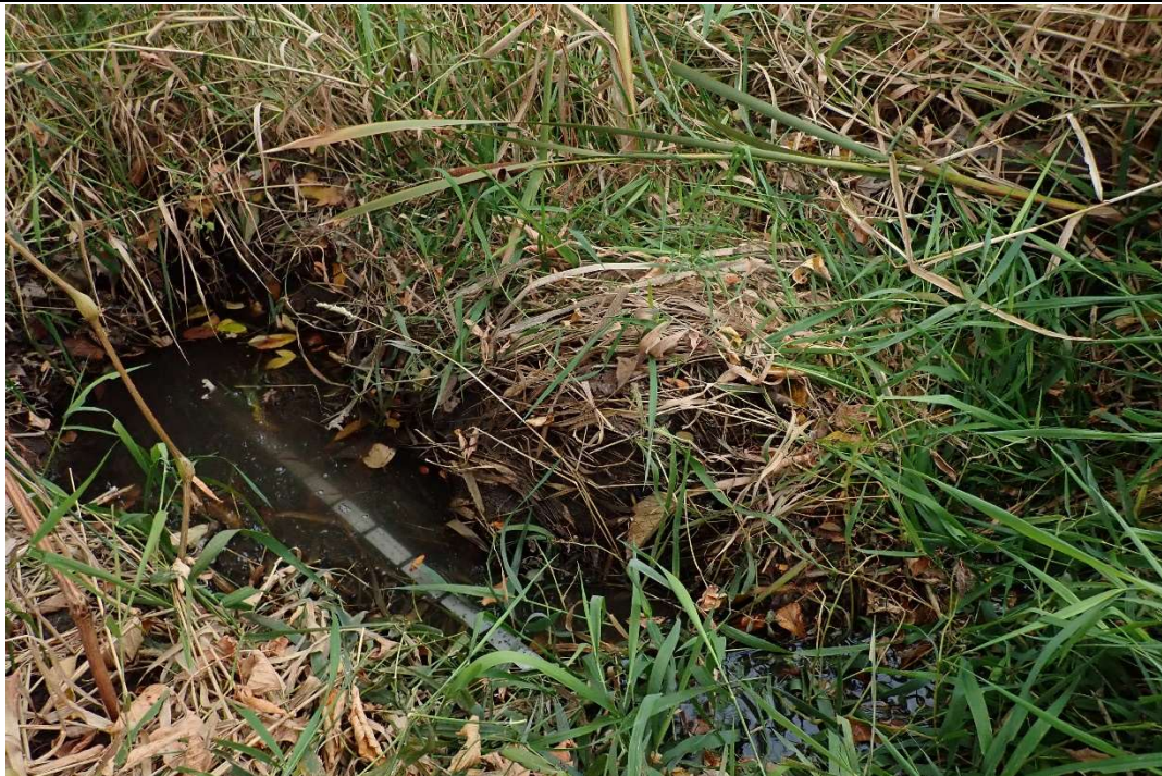
Defined bankfull conditions downstream of culvert. Metre stick for scale.
