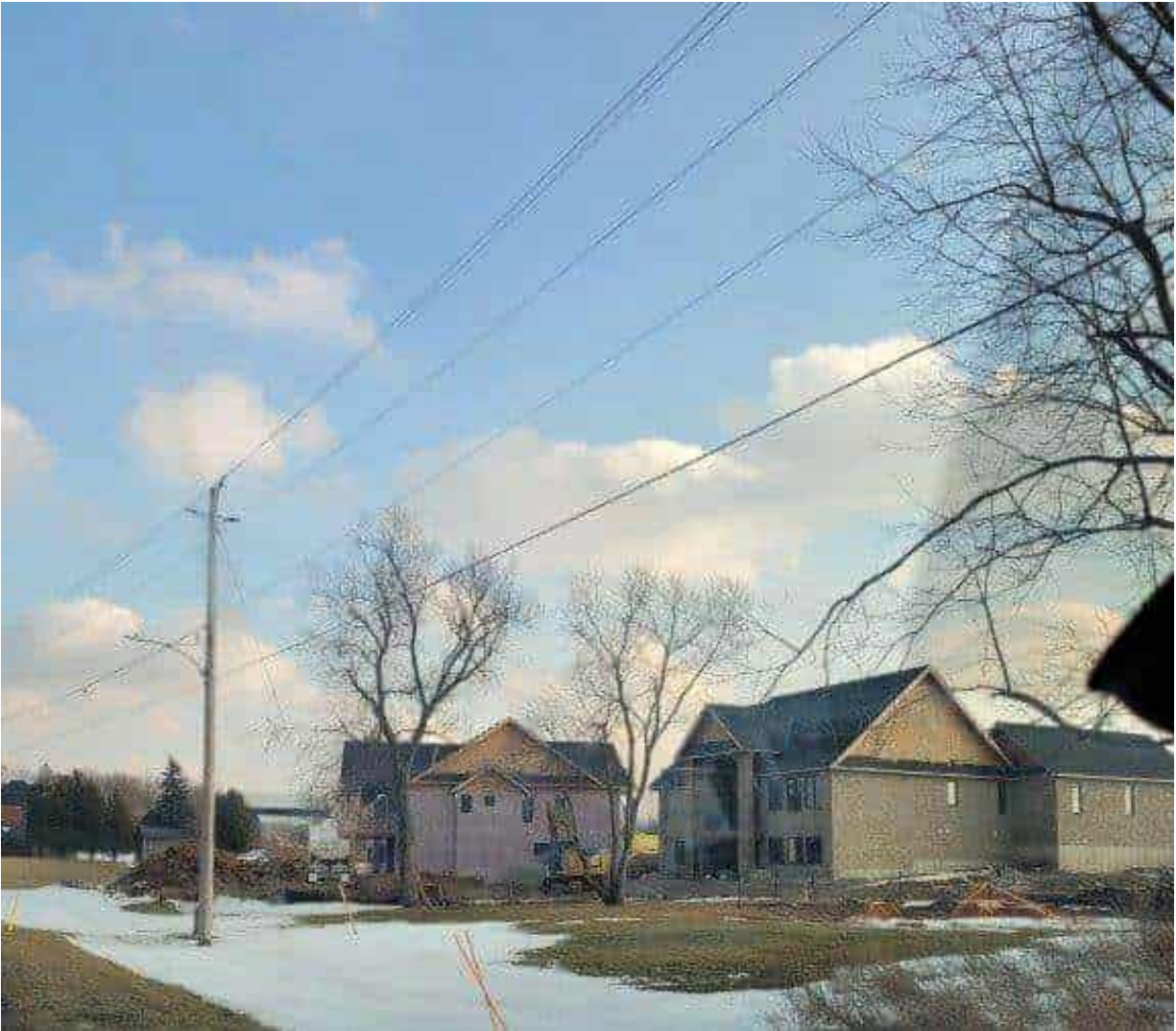
Photograph No 9. – South of study site, new construction residential neighbourhood.
