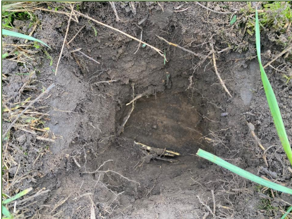
Photo 13: Typical Test Pit Facing North
