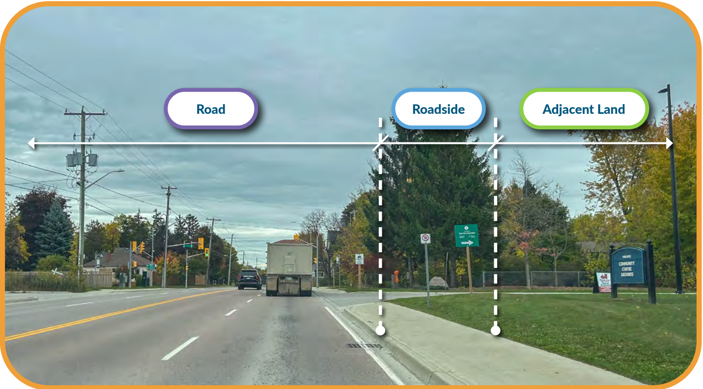
Heading south on Brock Rd S / WR 46. Pictured: entrance to Community Centre Grounds on right.
