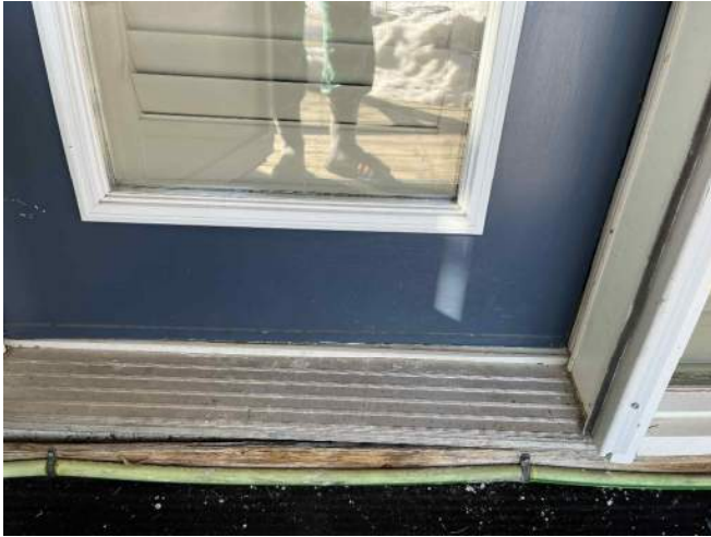
Basement Door – Outside
