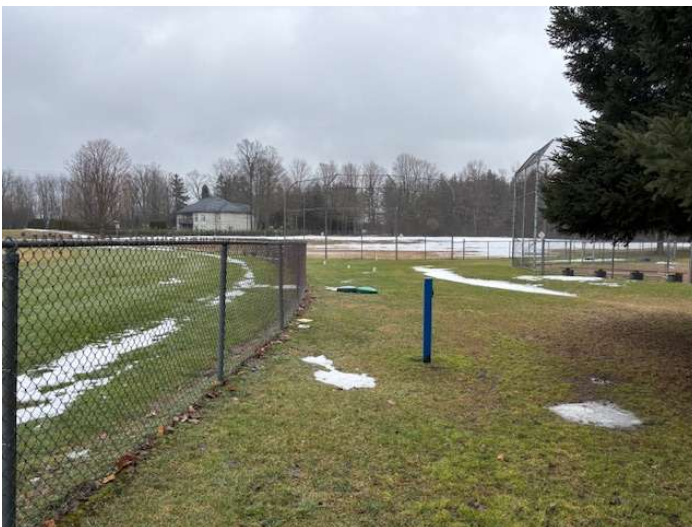
Figure 19 Additional shallow buried trench installed outside of fence line between play fields.
