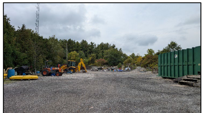
Image 19. Maintenance Yard and Waste Facility
