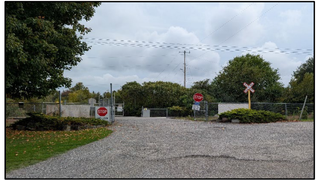
Image 18. Level Railway Crossing (Looking North)
