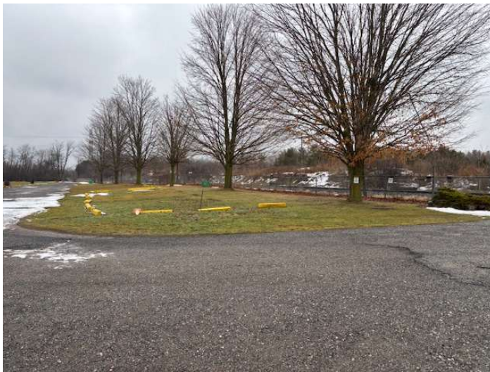
Figure 15 Disposal bed servicing water park field washrooms.
