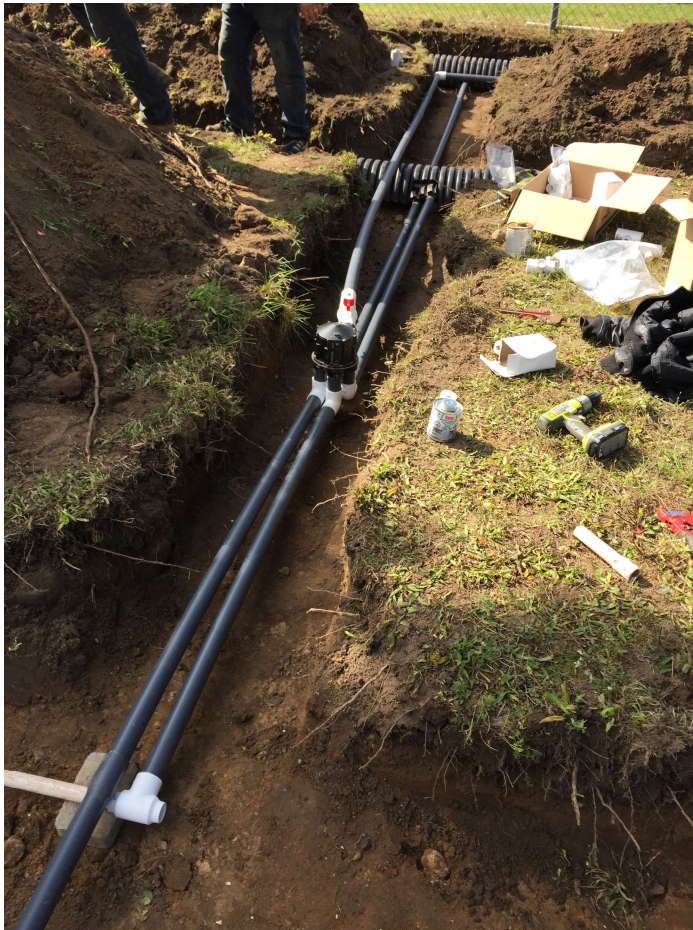
Figure 20 Installation of shallow buried trench disposal bed November 2015.
