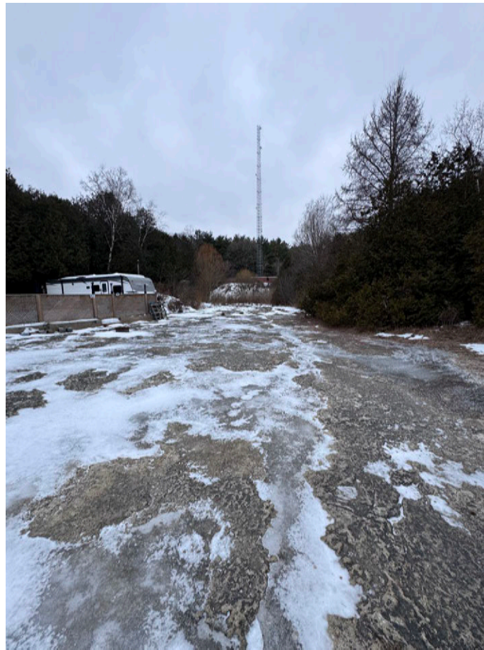
Image 5. Bedrock Area adjacent pond, looking west from southern limit of pond
